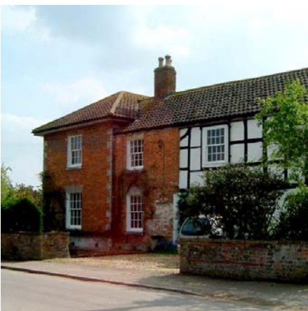
Townsend Farmhouse is typical of a number of buildings in Poulshot in that it has 17 th century origins with later alterations and extensions. The sash window within the timber frame section is probably 19 th century.
