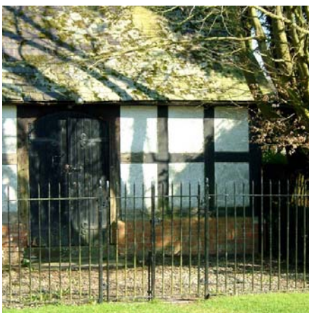
Attention to detail is important in any development within the Conservation Area. This can be seen in the construction of the building and retention of original railings at the former Church of St Paul.
