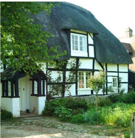
Surviving early buildings in Poulshot are timber frame with rendered panels or brick infill. Breastlands dates from the 16 th century. The thatch here is combed wheat reed but would undoubtedly have once been long straw.
