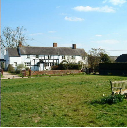
Timber frame and painted dwellings such as 51 The Green are more noticeable than those built in brick. No. 51 dates from the 17 th century with alterations and extensions of the 19 th century. The slate roofing was probably imported via the canal.
